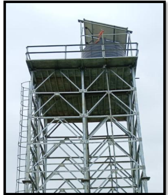
ELEVATED TANK PLATFORM & SOLAR PANEL MOUNTING — JJM SITE INSTALLATION, CHHATTISGARH
