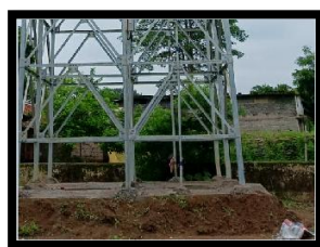
COLUMN BASE & FOUNDATION INTERFACE
