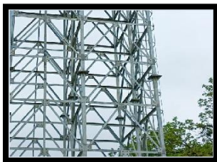
CROSS BRACING SYSTEM — HDG STEEL FRAMEWORK
